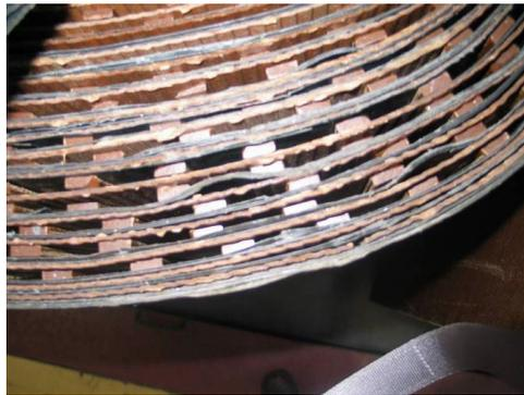
**Figure 1. Foil wound diamond dot winding**
