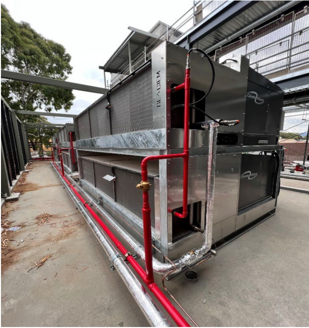
Figure 7 The three DP-CO 2 modules installed at Coles Norwood.
