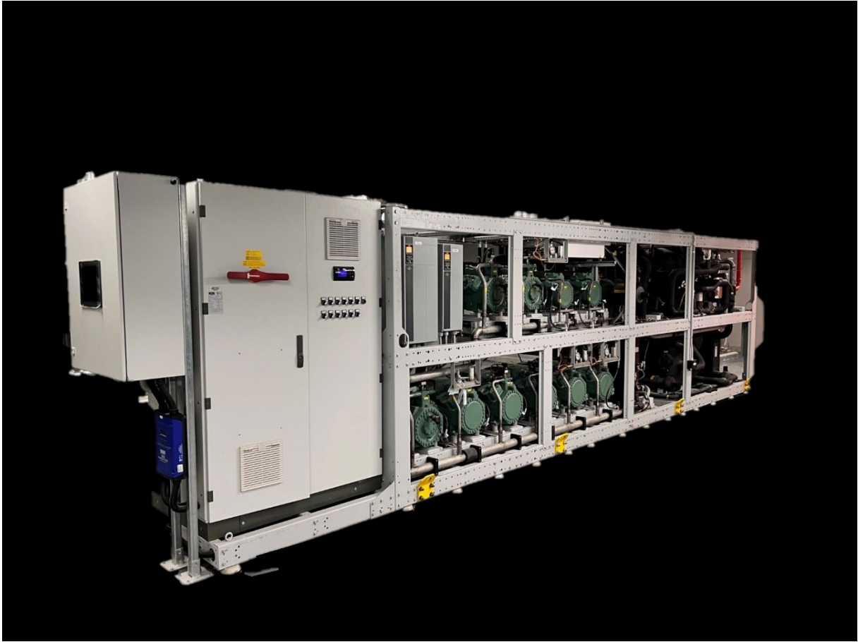
Figure 17 Plant room, Glaciem Electrical box with PLC, HMI attached on the left-hand side of the CO 2 Rack.
