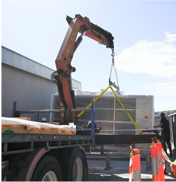
Unloading the Rheem RTHP540 heat pump system for installation.
