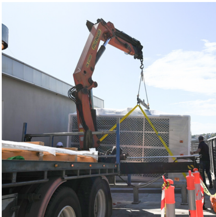
Unloading the Rheem RTHP540 heat pump system for installation.
