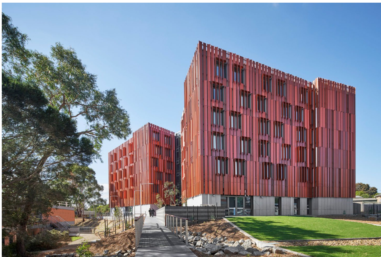
Figure 9. Gillies Hall, Monash University. This new student accommodation complex at Monash University's Peninsula campus uses a Passive House-certified design that greatly reduces energy consumption. (Source: Jackson Clements Burrows Architects, Photographer: Peter Clarke)
